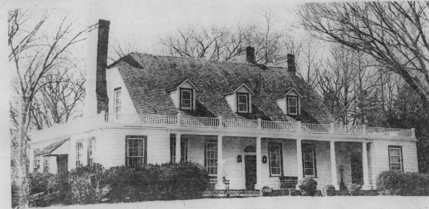
RIPPON LODGE—This house was built by Colonel Richard Blackburn in 1725 and is said to be the oldest home of note in Prince William County. The veranda commands a sweeping view of Neab-
